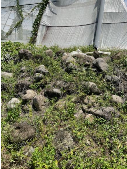
Figure 9 (Left) The first attempt to stabilize the area next to the new greenhouse involved placing large rocks on the slope. This method was too labor intensive and did not work.
