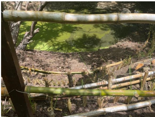
Figure 19 Vetiver securing the banks of a newly created rain pond in the High North established to support diverse animals in the area
