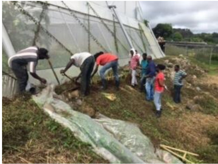
Figure 9 (Left) The first attempt to stabilize the area next to the new greenhouse involved placing large rocks on the slope. This method was too labor intensive and did not work.
