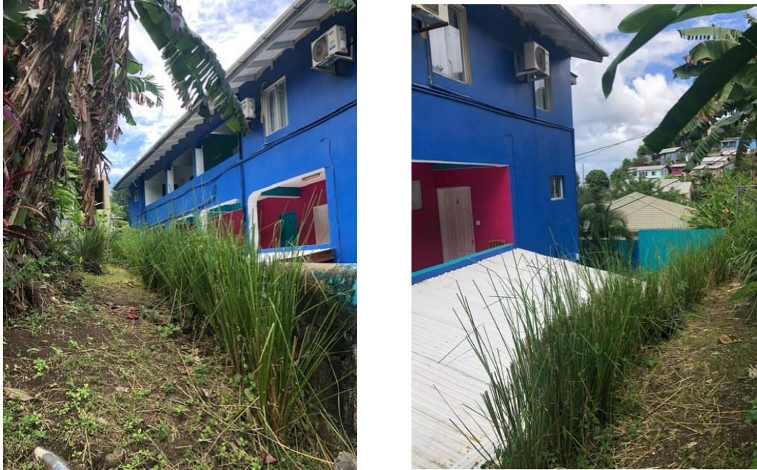
Figure 16 Images of Vetiver hedge stabilizing hillside above Sea Breeze hotel in Grand Anse
