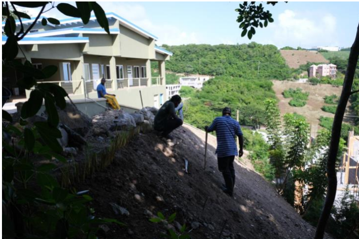
Figure 17 Images showing VS demo installation in Nov 2020 on very steep bare slopes on a housing site (image provided by J. Barcant). Followed by a photo taken in July 2021 showing well established vetiver hedges stopping significant soil erosion and slope slippage.
